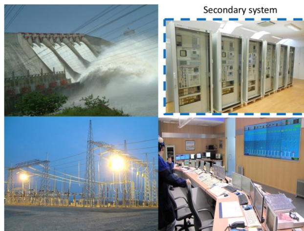
Figure 1 Secondary systems made by CCE
